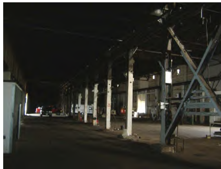
Photograph 12 - Interior of central section of building.
