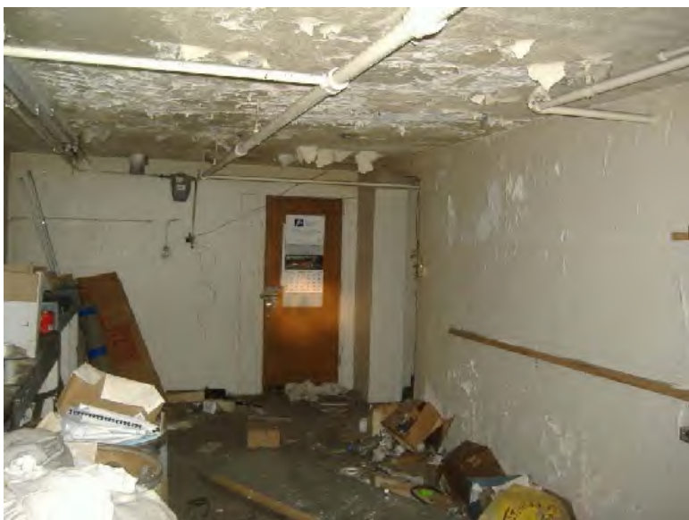
Photograph 11 - Interior of Property building.
