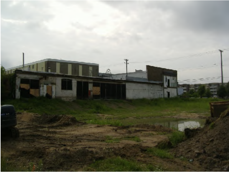
Photograph 5 - Subject property (view to the southeast from 29 th Avenue SE). Foreground is area of demolished section of building that is now part of the light rail project.
