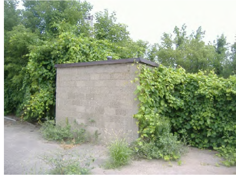
Photograph 6 - Shed in northeast corner of Property.
