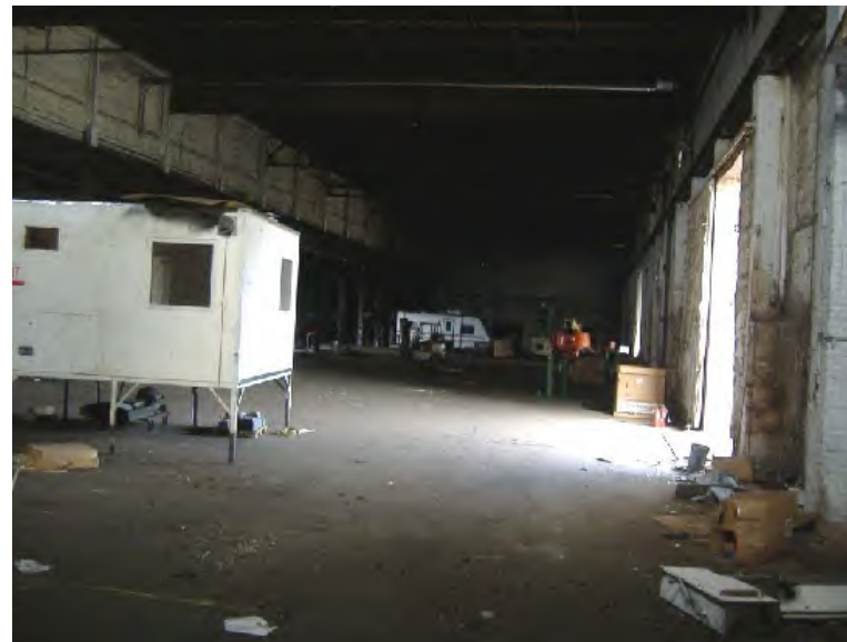
Photograph 10 - Interior of central section of building.
