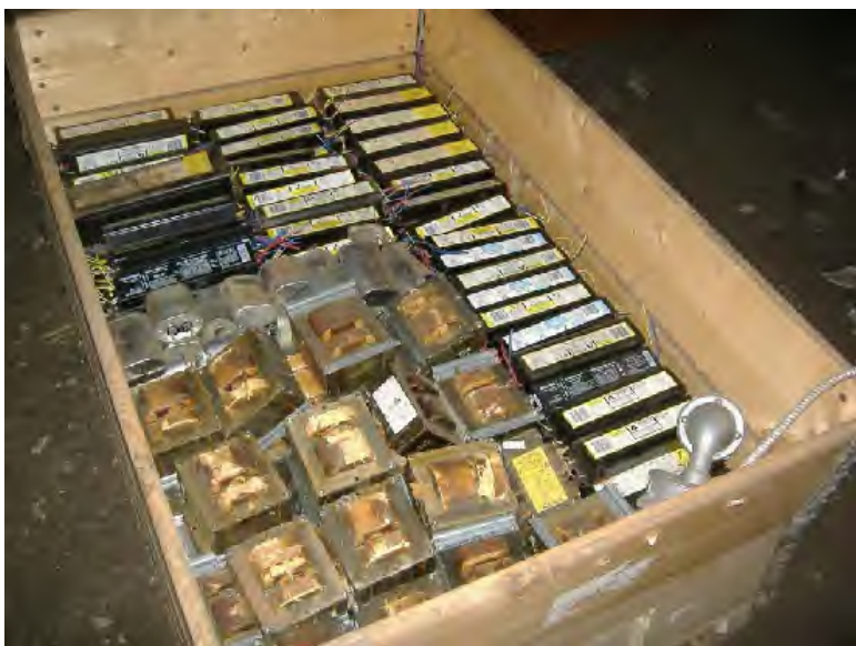
Photograph 15 - Switches and fluorescent lamp ballasts storage.
