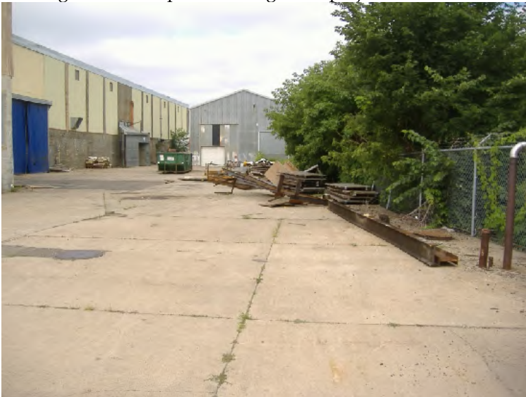
Photograph 7 - Yard of Property with manhole covers, fill and vent pipes associated with USTs in foreground (view to west).
