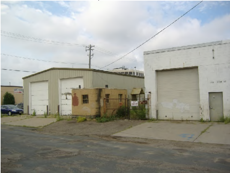
Photograph 3 - East end of Property building.
