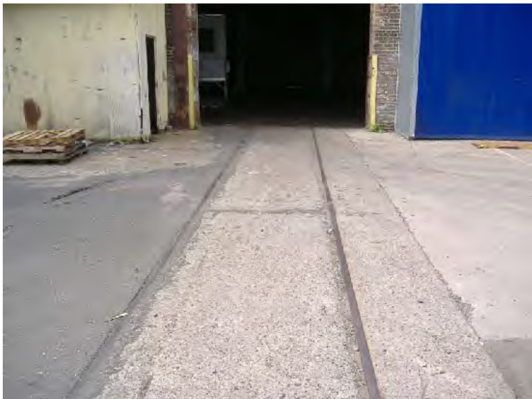
Photograph 9 - Tracks entering Property building.
